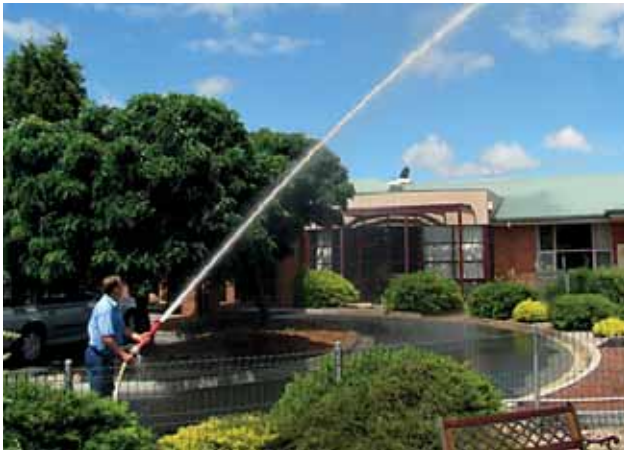
Simon Healy testing fire hoses
